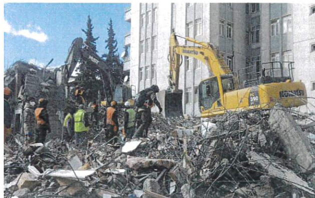
On 15 February 2023, PIAHC offered assistance on a new site to retrieve the remains of 3 persons.
