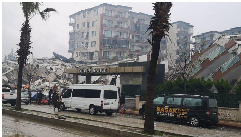
The Guclu Bahce complex in Antakya. Credit: BBC News
