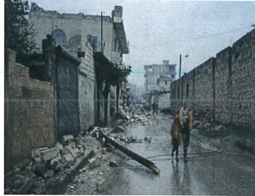
Mother and child walked hand-in-hand next to collapsed houses in North-west Syria. 8 February 2023. Credit: OCHA/Mohanad Zayat
